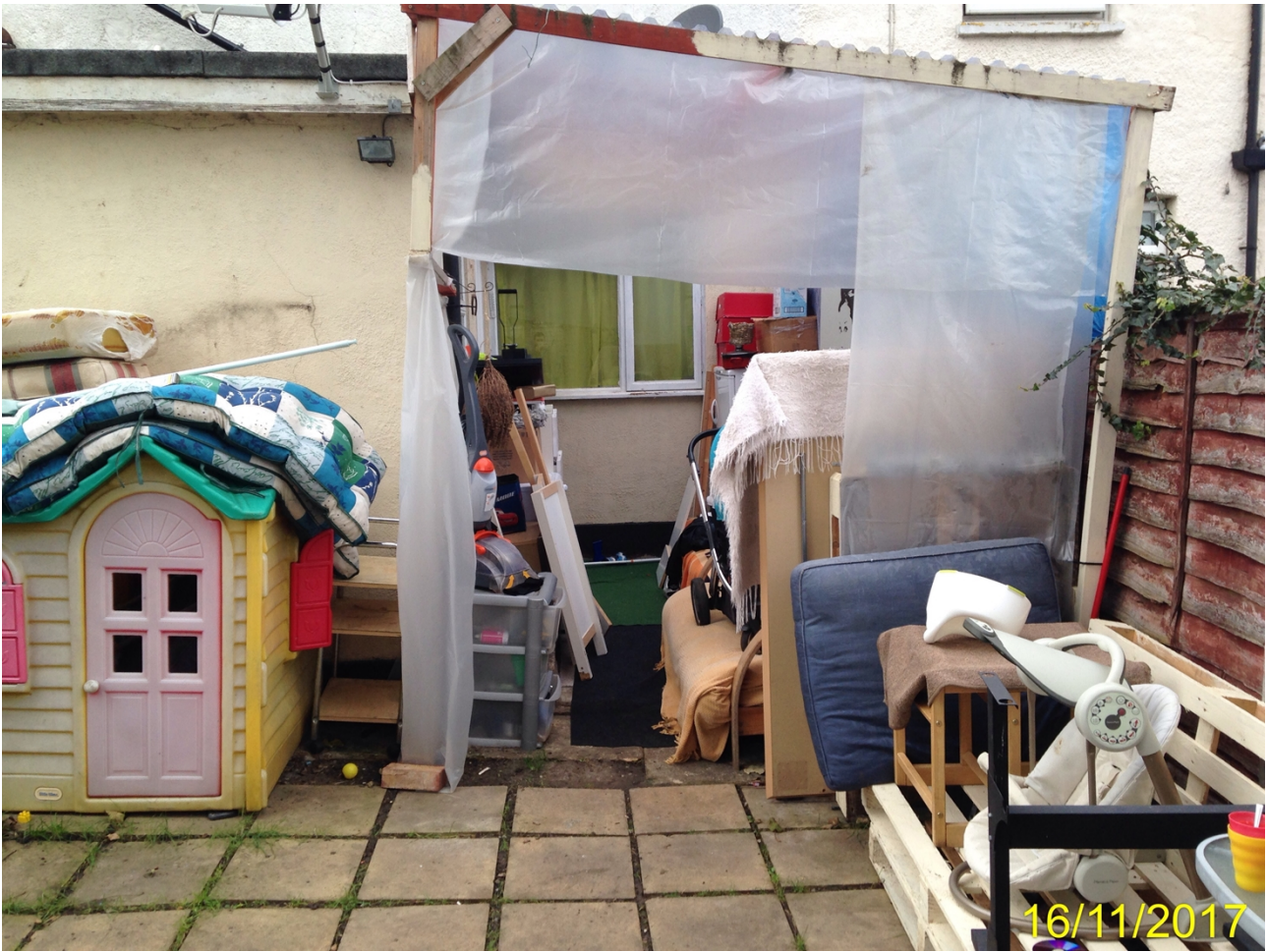
View of unlawful extension from rear garden
